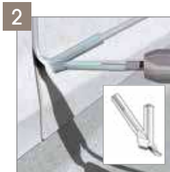
Perfect CR 41 wall weld - H231
